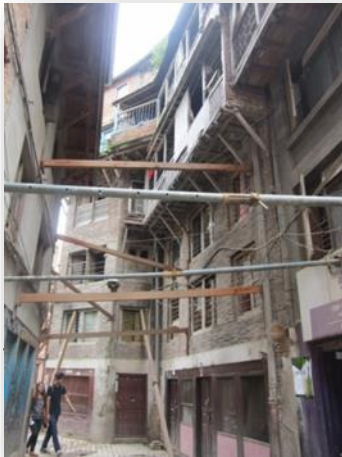
Temporary pillars with old houses
