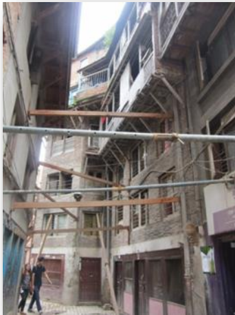
Temporary pillars with old houses
