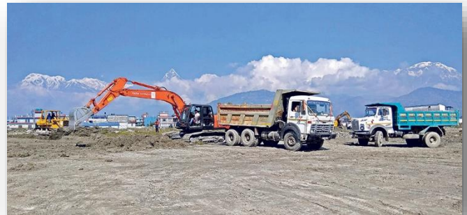
New Pokhara International Airport
