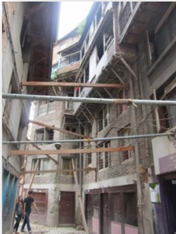
Temporary pillars with old houses
